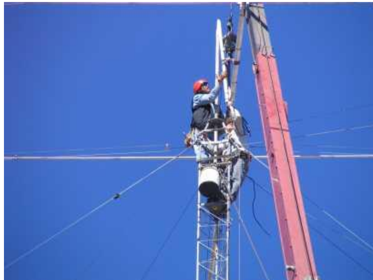
Putting up the two 4L40 Yagis at N6RO with big crane.
